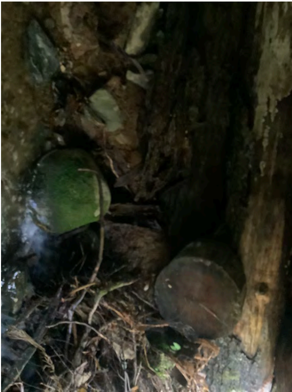
Right Bank Abutment when facing downstream
